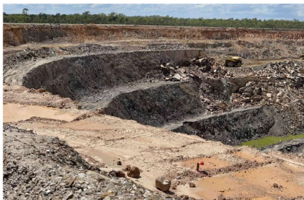
The Open Cut at the official opening of the Finnis Lithium mine Picture: Glenn Campbell
